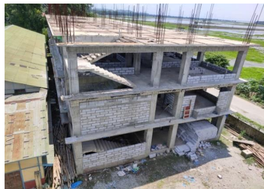
Figure 2. 14. New Laboratory building under construction
