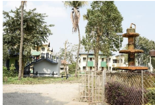
Figure 2. 12. Water treatment plant
